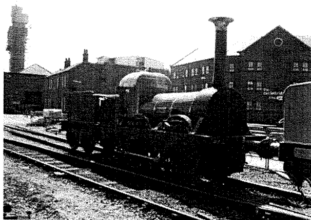
With the towbar attached to the 'eye' on the front of 'Lion', the locomotive could be gently moved outside the power hall. The improbable structure in the left background is set to become Manchester's tallest office block.
